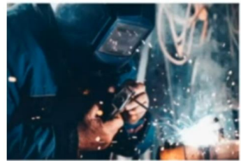
Welding - joining metal
